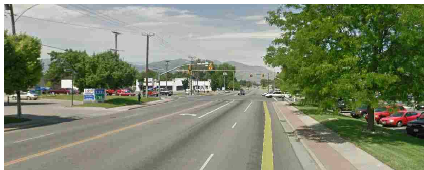
Figure 1: 3500 South / 5600 West intersection, looking to the west (Google).
